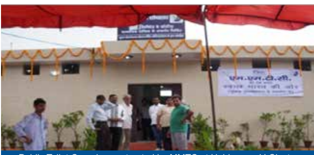
Public Toilet Complex constructed by MMTC at Haiderpur, JJ Cluster
