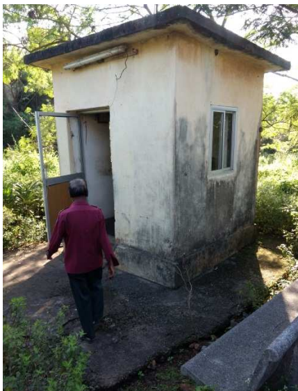
Existing security cabin near entrance
