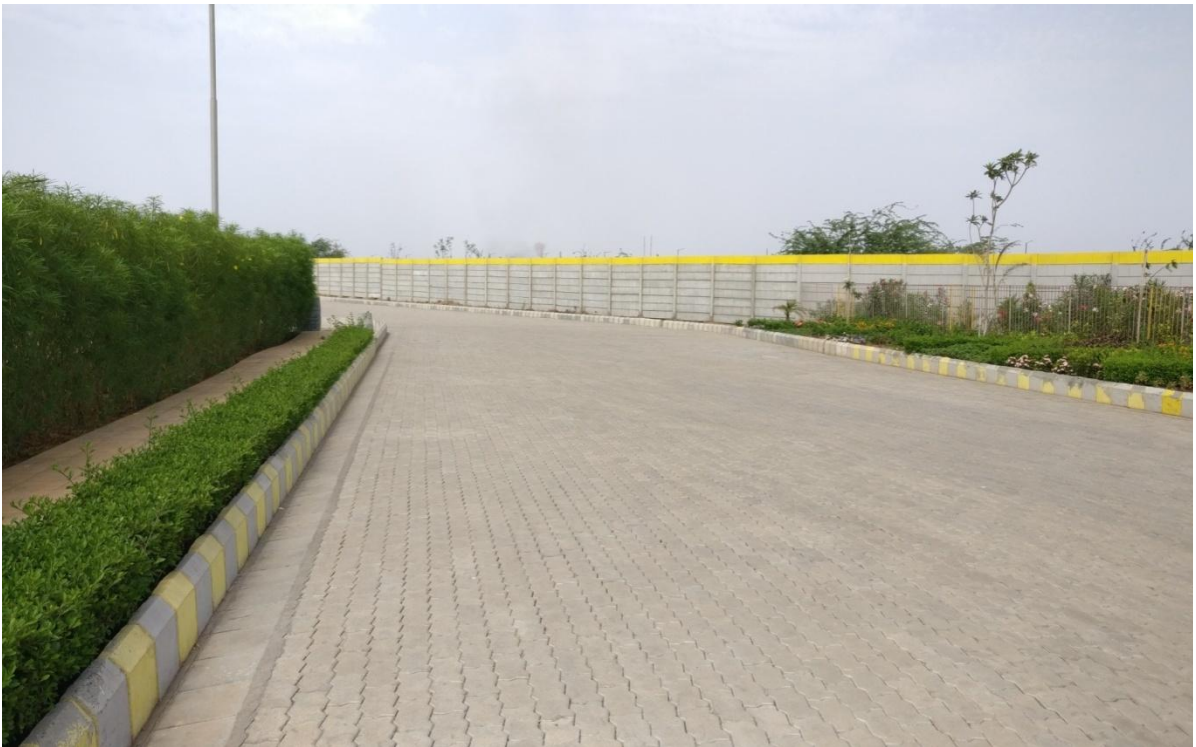
View of Paved Road (Partially Completed)
