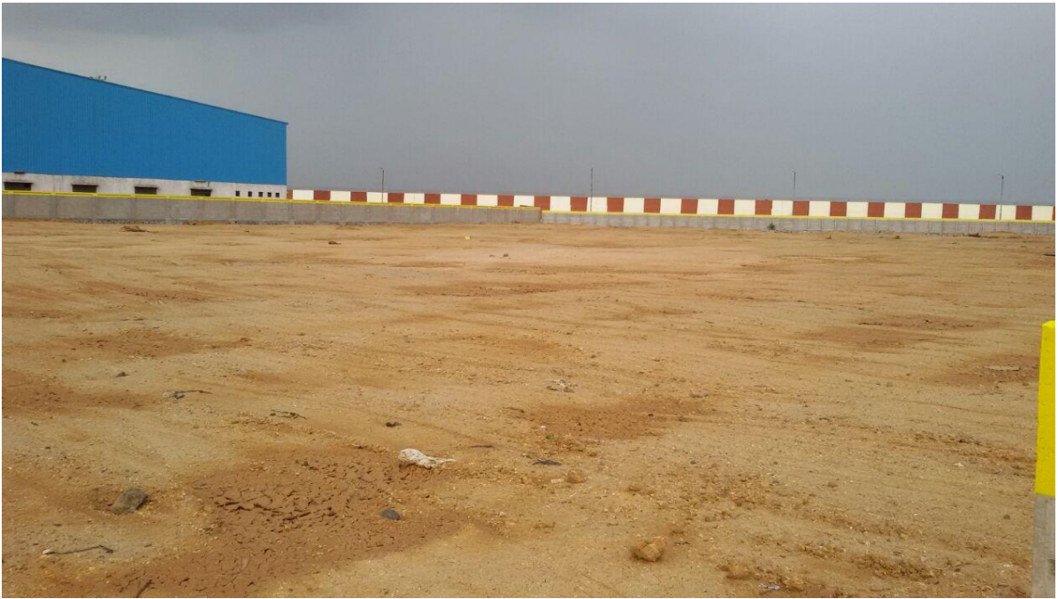
View of Levelled Ground subsequent to Cutting & Filling (Partially Completed)
