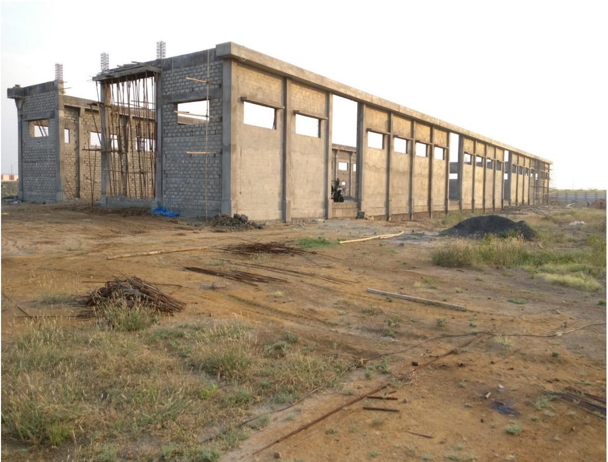
View of Warehouse (Partially Completed)
