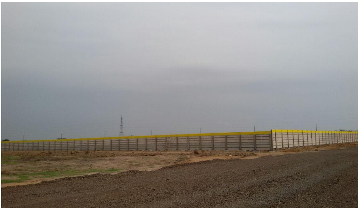
View of completed boundary wall
