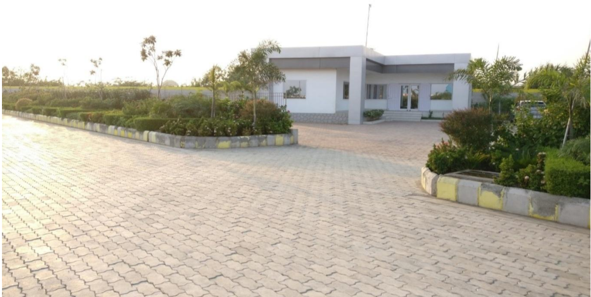
View of Common Facility Centre (Completed)
