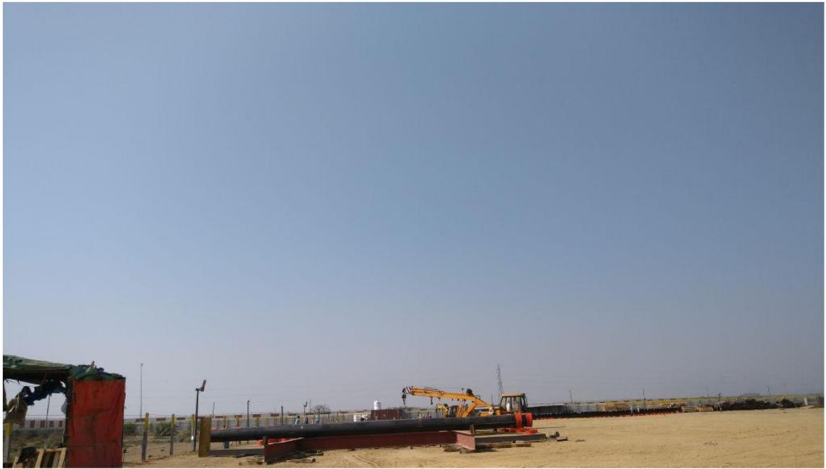
View of Open Warehousing for Pipes (United Drillings)
