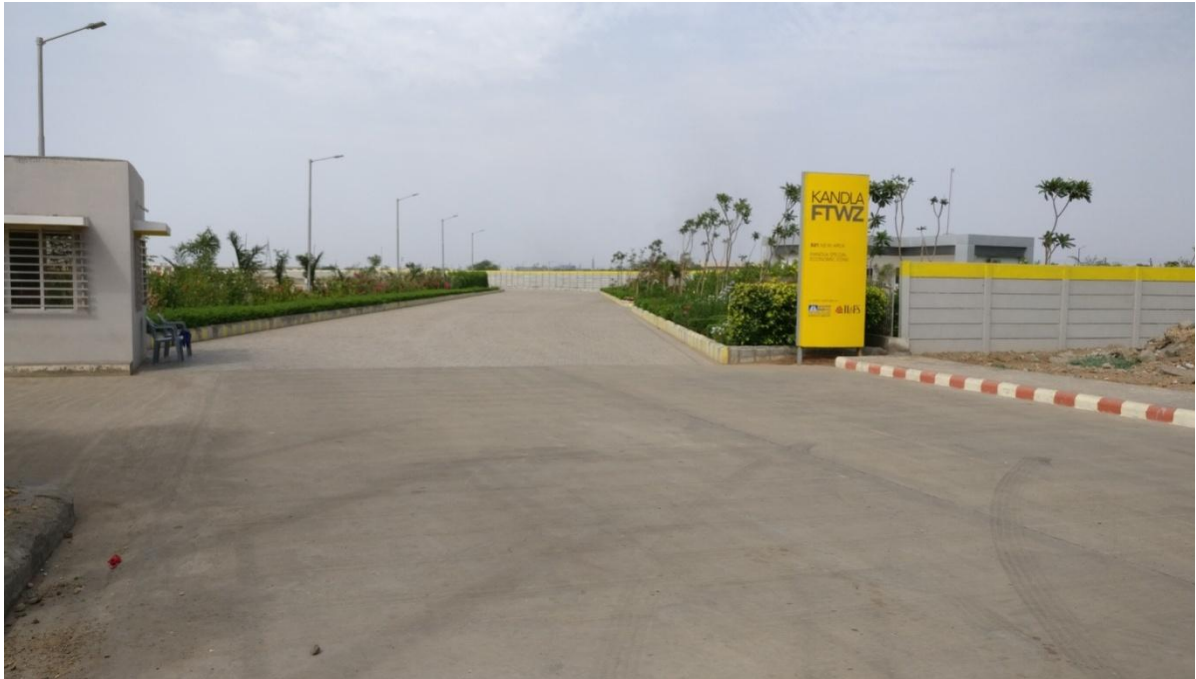
View of Entry Gate (Completed)
