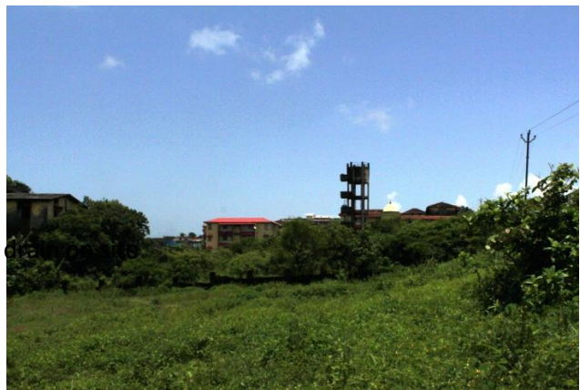
Overhead water reservoir exists on site
